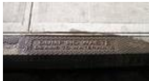
Dump no Waste Drains to Waterways
