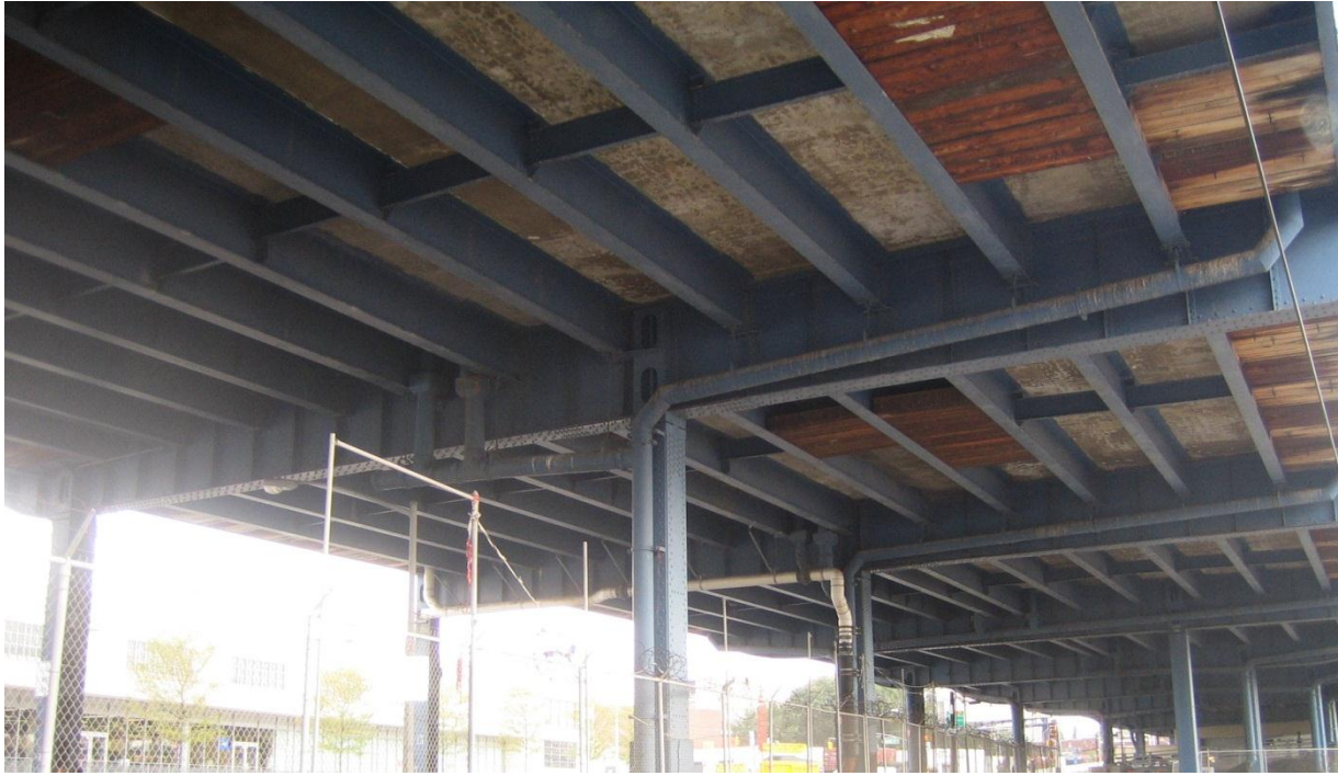
Drain pipes go across more than six lanes.
