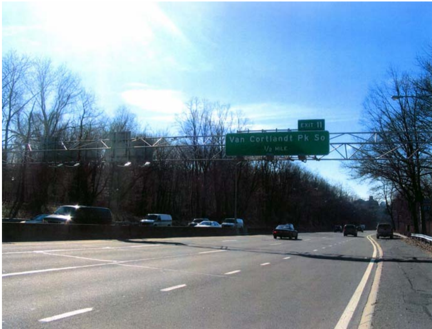
Figure 3-15 Major Deegan Expressway Existing Sign in Van Cortlandt Park
