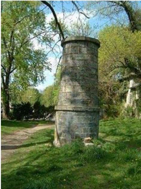
Figure 4-6 Old Croton Aqueduct Ventilator
