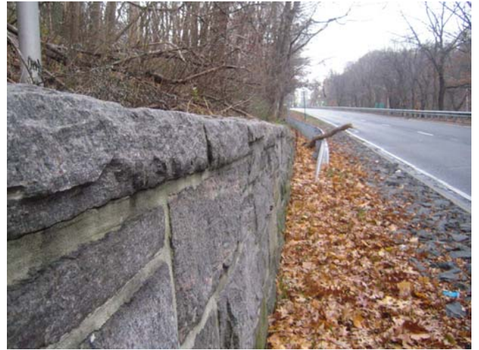
Mosholu Parkway, beginning of retaining wall (looking south)
