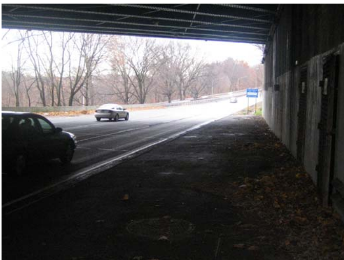
Mosholu Underpass, shoulder (looking north)
