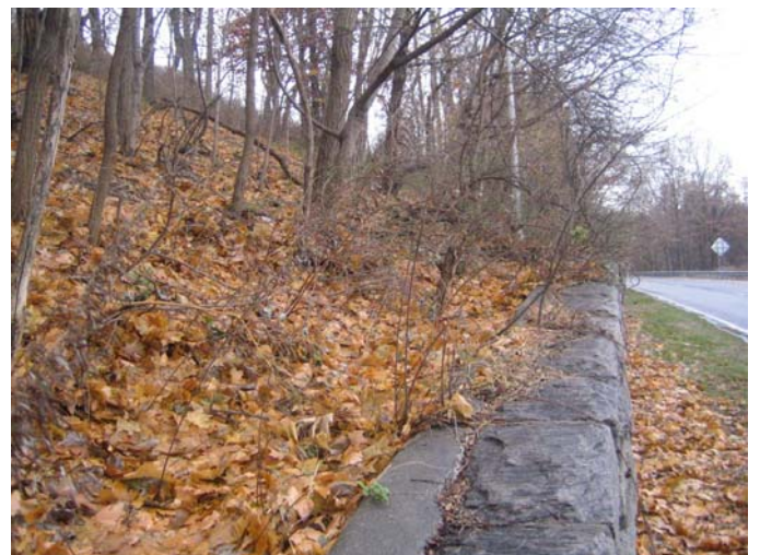
End of the retaining wall at the Mosholu Underpass (looking south)
