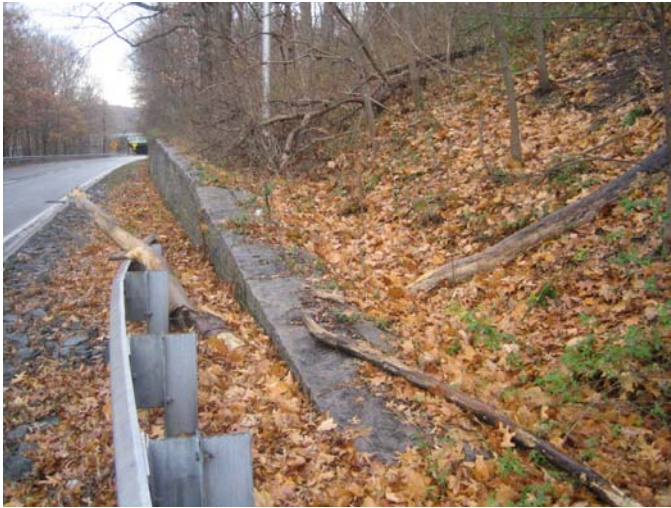
Mosholu Parkway, beginning of retaining wall (looking north)
