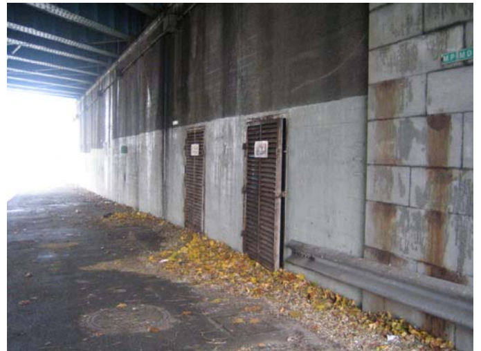
Mosholu Underpass, shoulder
