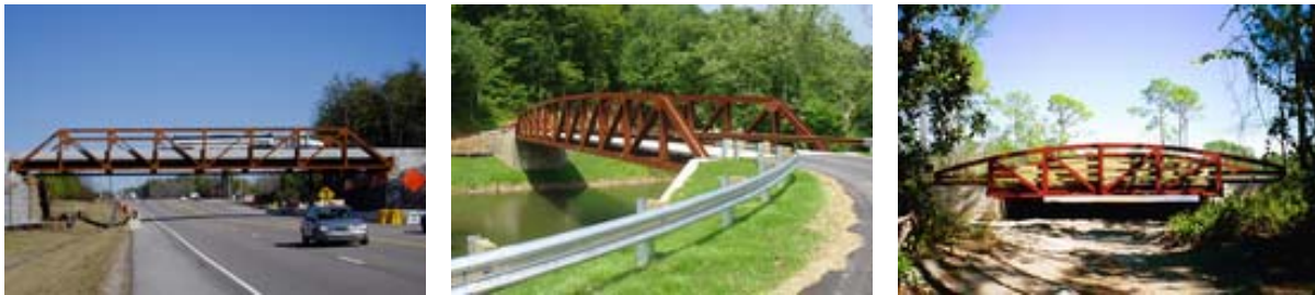
Figures 3-17 Examples of Metal Truss Bridges
