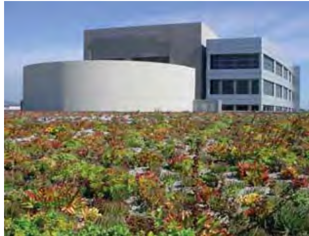
The green roof at Ford Motor Company's Premier Automotive North American Headquarters in Irvine, CA, was designed to visually mimic the natural landscape. PHOTO COURTESY OF ROOFSCAPES, INC.
