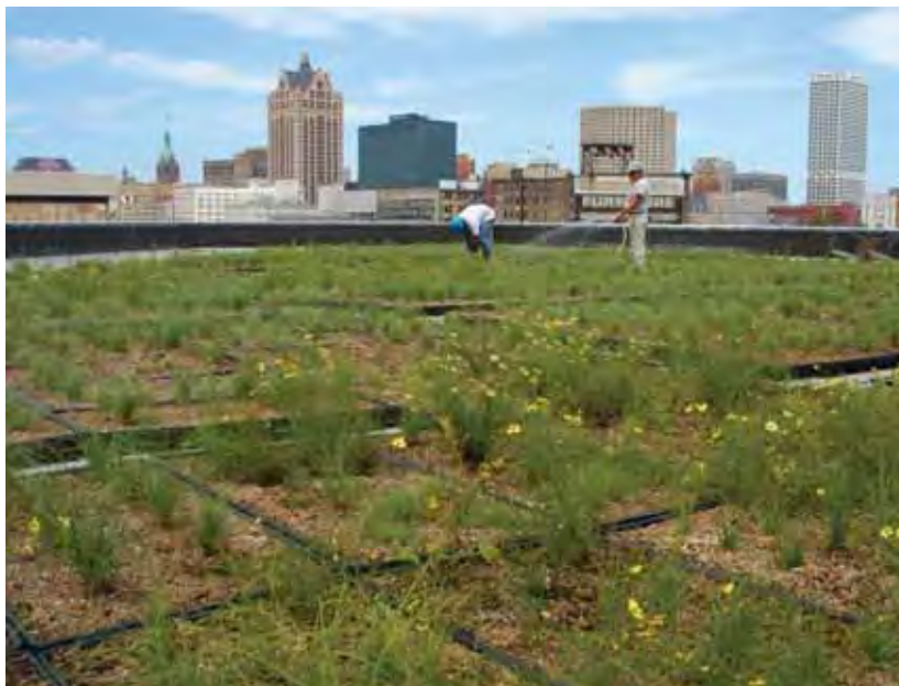
The green roof atop MMSD's headquarters, shown just after installation, demonstrates how stormwater flow into the city's sewer system could be reduced.
