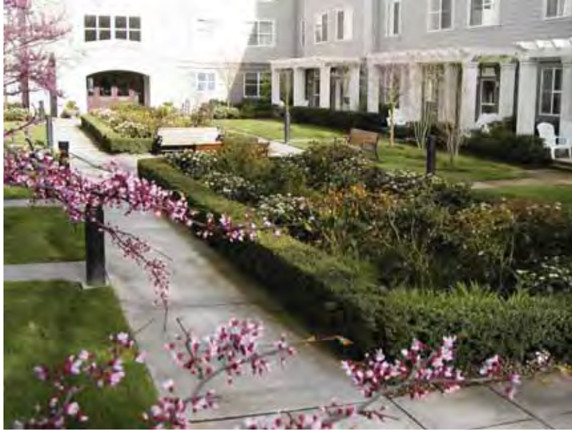
The vegetated infiltration basins in the Buckman Heights Apartments courtyard in Portland, OR, receive and infiltrate stormwater from building roofs and sidewalks.
