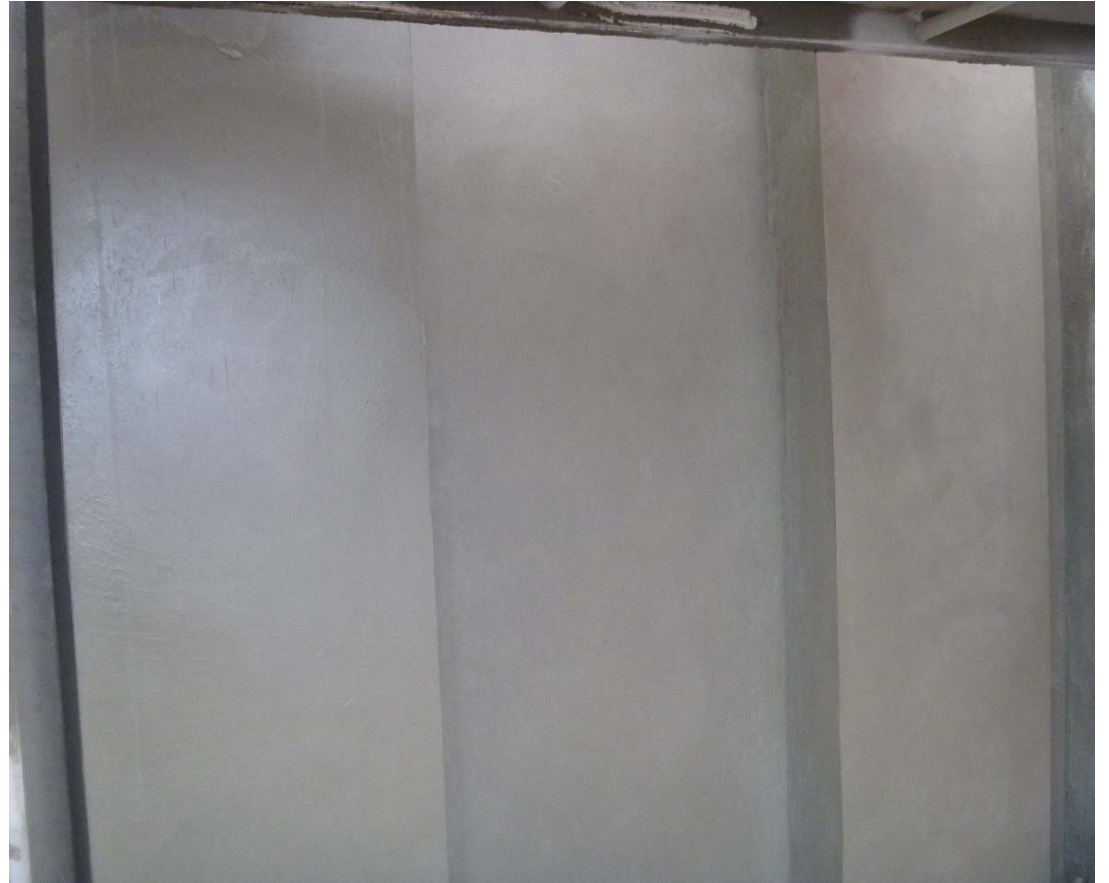
Shotcrete Troweled Finish Example: East Side Access Tunnel, Manhattan October 2015
