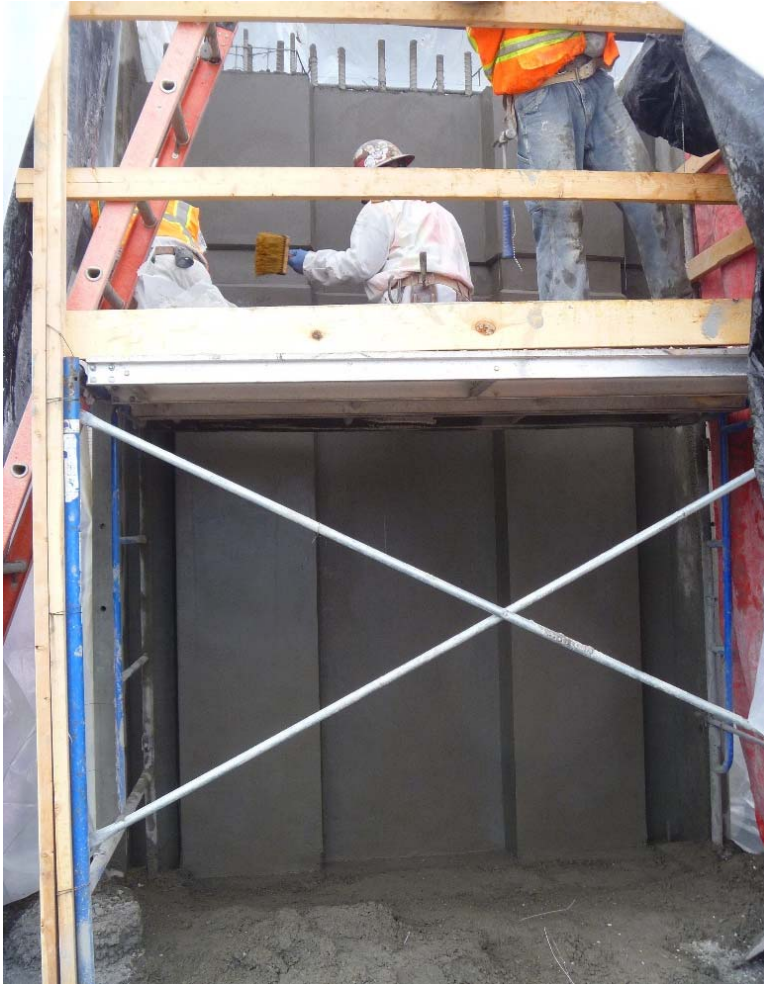
Shotcrete Troweled Finish Example: East Side Access Tunnel, Manhattan October 2015
